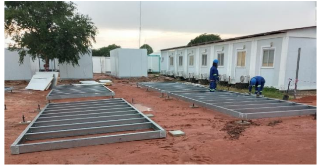
Figures below: Early stages during installation of accommodation units
