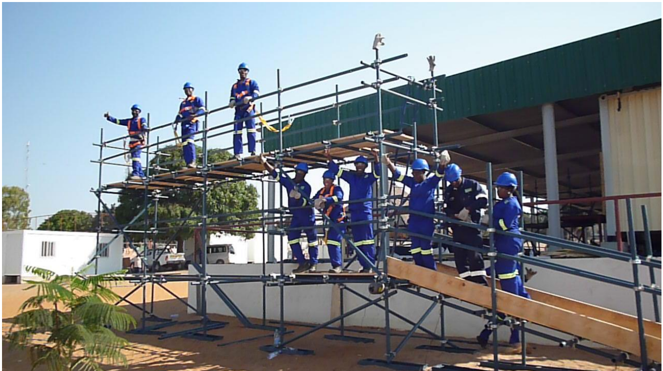
Above: Futuro Skills Mozambique students undergoing scaffolding training.
