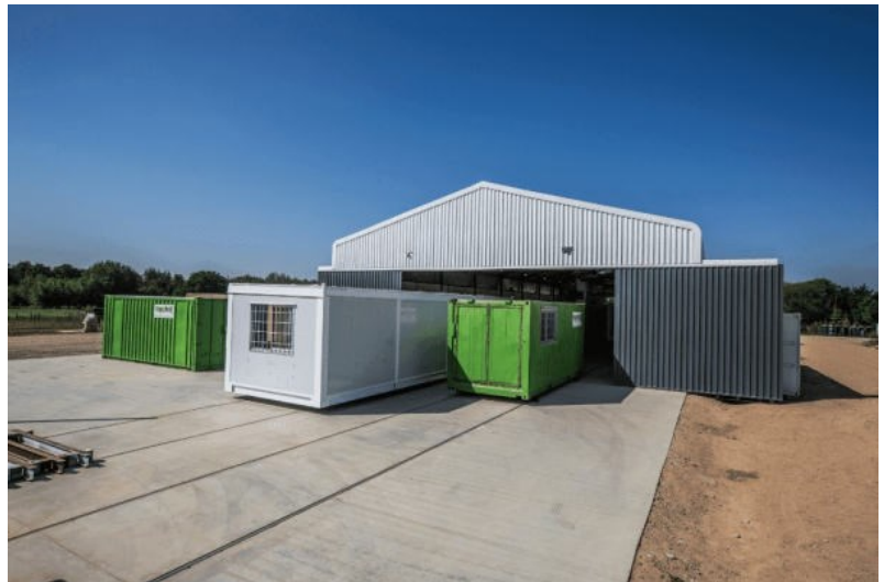
Figure 5 – Example of MBA Facility
