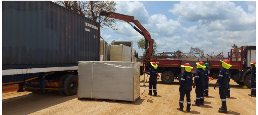
Mobilisation of equipment – WBHO Site
