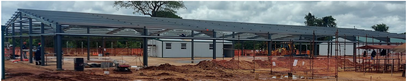
Mess Hall and Service facility Steel Structure
