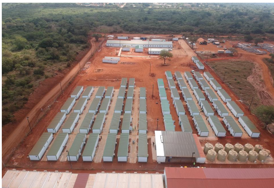
Above: TSK 420-man camp with support facilities near ready for handover
